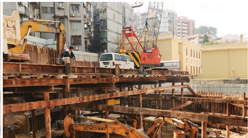
Excavation and lateral support works were recently completed at The Fountainside
