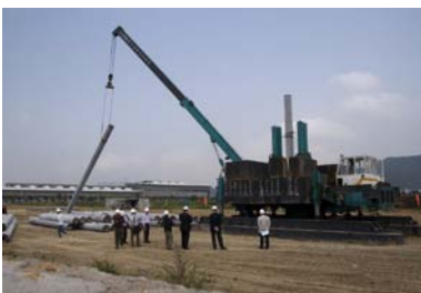
The development phase has commenced, with foundation works currently underway.
