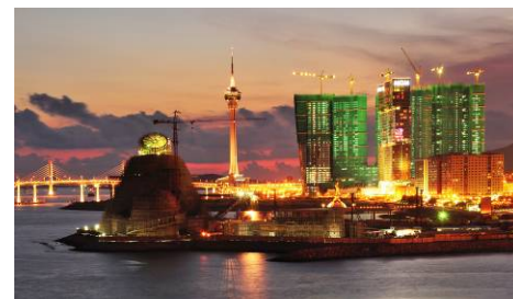
One Central, scheduled for completion in late 2009, occupies an unprecedented location on Macau Peninsula.
